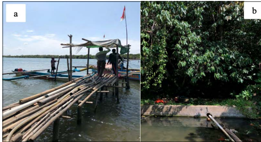
Figure 3. Piped water supply for Nusakambangan Island springs: (a) Pipes to the boat to collect water (b) pipe source with pump
